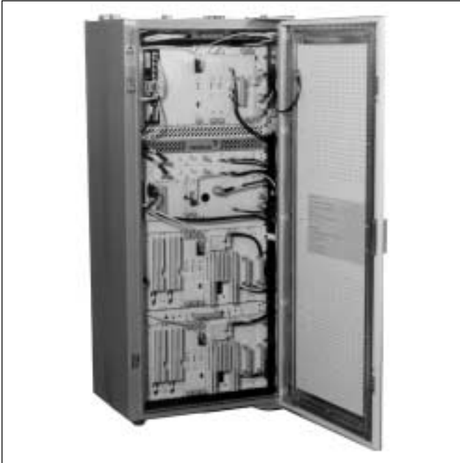
Base station of cellular network
